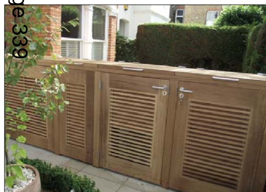
TIMBER REFUSE AND CYCLE STORAGE ENCLOSURE
